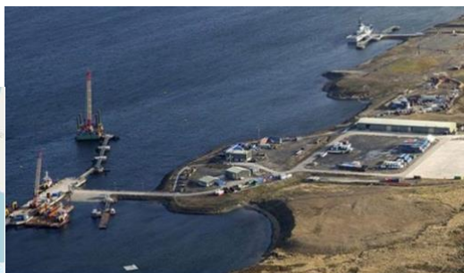
The new facility will enable larger 20,000 tons Point Class vessels to berth in the harbor, delivering military
